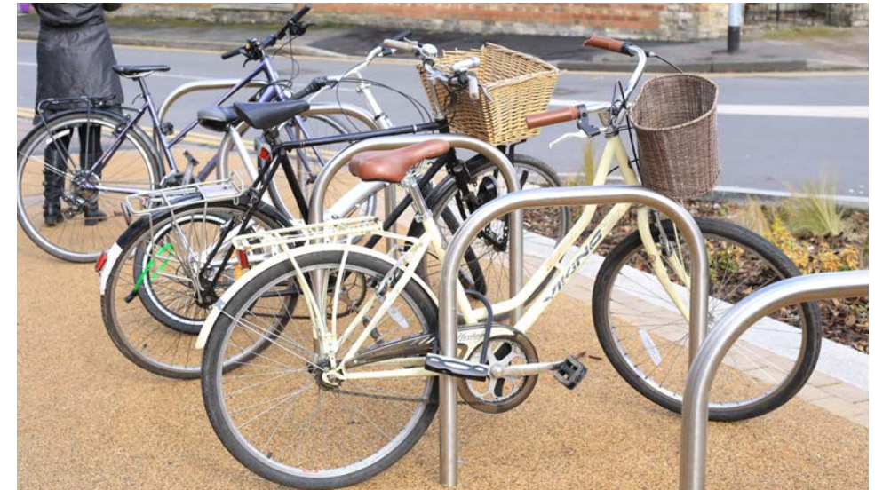
Well designed cycle parking in public realm (Sheffield stands)
