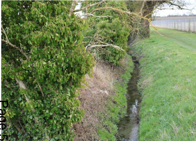
① Existing ditch and vegetated bank
